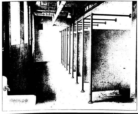
These Lavatory **Partitions** are made of Galvanized Steel Framing, Wrought Iron Pipe and Steel Angles.
