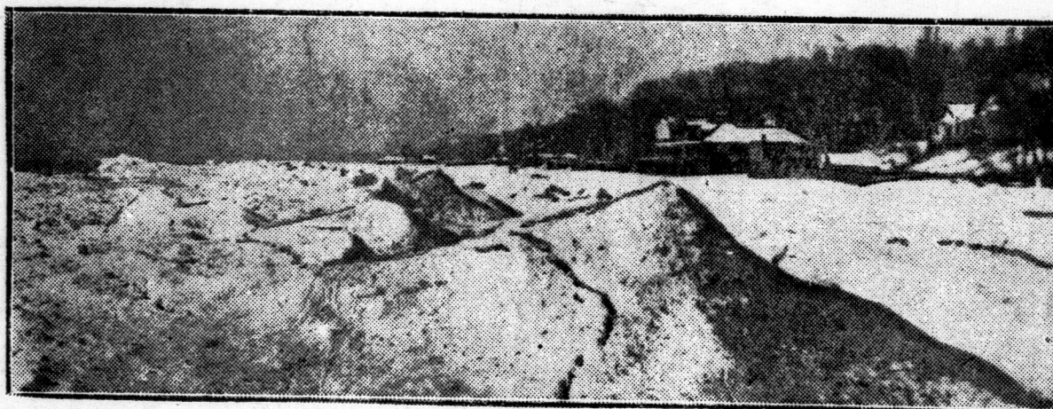
First signs of spring. The ice on the Toronto lake front is already beginning to crack and break up.
