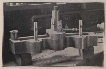
Fig. 8. Locating the Saddle Correctly on the Link.
