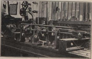
Fig. 9. Machine for Finishing the Tumbling Shaft Arms.
