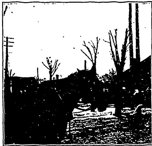
Maple Trees Butchered to "Clear" Wires Overhead
