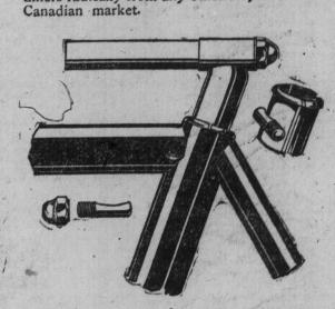
The working principle of this seat post fastener is shown in the accompanying illustration. The cotter key, milled away on one side to fit over expanding ring, is tightened so as to give the friction required to hold the seat post securely.
