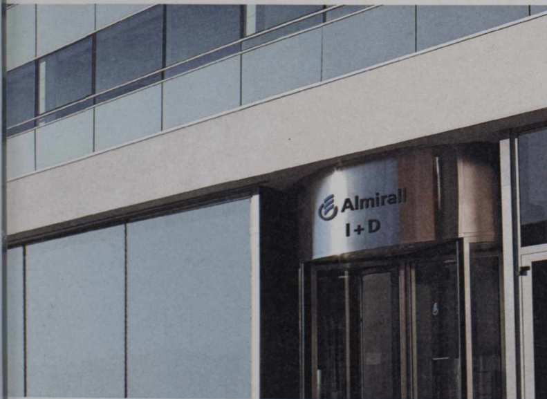
Almirall Sant Feliu R&D centre in the outskirts of Barcelona (Spain)
