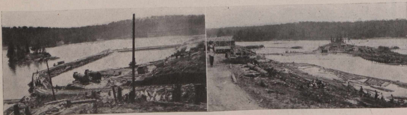
Fig. 4.—Cofferdams Above and Below the Falls Before Dewatering the Power House Site.
