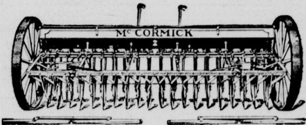
A McCORMICK drill, used to plant the seed in your fields, will bring extra dollars into your pockets at the next harvest. It will deposit the seed at the right depth to secure sufficient moisture and plant food, and to give the seed the best kind of a start.
