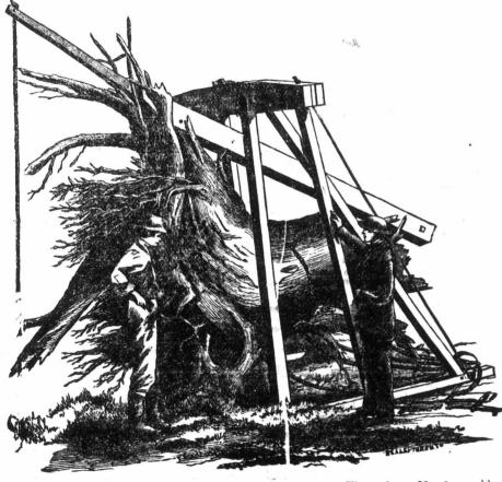
Will take out 20 to 50 stumps per day, depending on size. Three sizes. No. 1. capable of drawing any stump, \$129. No. 2, for stumps 2 feet 6 inches. \$99. No. 3, for 18 inch stumps, \$70. The largest sizes will take out the smallest stumps, but they are constructed much stronger and heavier.—Apply to PLUMMER & PACEY, Waggon Makers, London, or to W. WELD, Agricultural Emporium.
