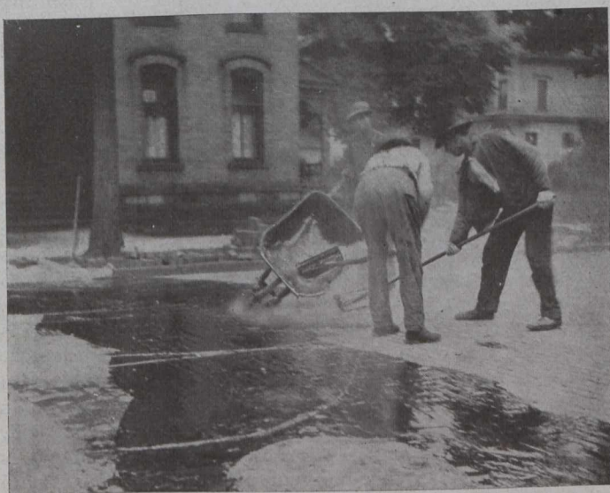
Fig. 1.—Finishing Mastic Filler on Brick Pavement.
