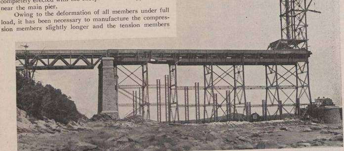
Fig. 2.—Falsework and Floor Erected, and a Start Being Made on the Erection of the Main Shoes.
