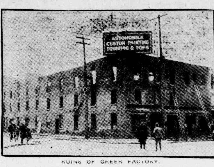
RUINS OF GREER FACTORY. Ruins of the A. B. Greer & Son Company, which was almost completely destroyed by fire at an early hour this morning. The above picture was taken by an Advertiser photographer while the ruins were still smoldering. The interior of the structure was almost entirely destroyed, the four walls remain upright with little support. The loss is estimated at from $75,000 to $100,000.
