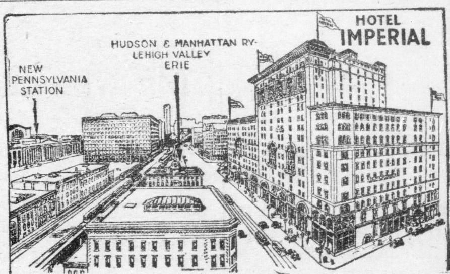
One Block from New Pennsylvania Station.
