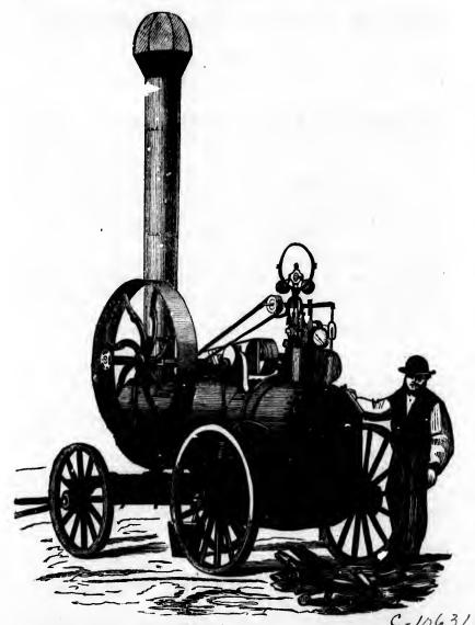
The above engraving represents my New Patent Portable Steam Engine, designed to meet a want long felt in Canada. This engine is adapted for driving a Threshing Machine, Shingle Machine, Grain Crusher, Sawing Wood, or any conceivable purpose requiring steam power. Being mounted on wheels, it is easily removed from place to place. Weight 4700 lbs., all complete.
