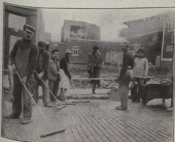
Fig. 2.—Applying Cement Grout Filler at Outremont, P.Q.
