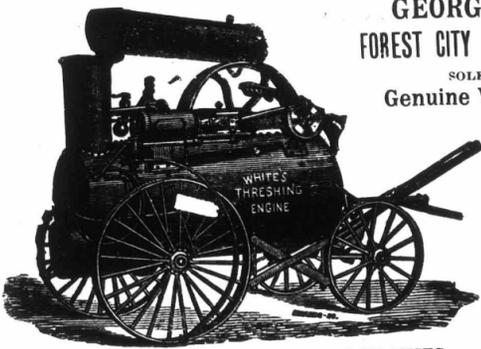
For wood or straw. Our Straw-burning Engine has given thorough satisfaction. It is the only straw-burner with back water space in boiler. **Light and Heavy Traction Engines, Special 16, 20 and 25 H. P. Semi-Portable Engines,** strong and compact for saw mill purposes, same style as our Threshing Engines. We can supply at any time Engines and Boilers, from 5 to 30 H. P., suitable for brick and tile yards, cheese factories, cider mills, saw mills, planing mills, etc.
