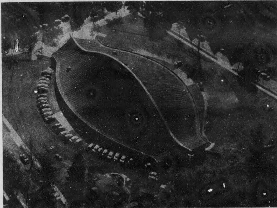
Above is pictured the David S. Ingalls Rink of Yale University, which will be host to the Devils on January 2, 1961. The whale-like structure seats approximately 2300 and cost in excess of one million dollars. The concrete roof was originally designed to be self-supporting. However a structural failure made necessary the addition of strong steel supports in the interior. These additions hoisted the cost \$300,000.
