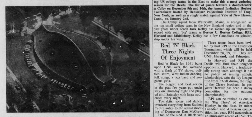
Above is pictured the David S. Ingalls Rink of Yale University, which will be host to the Devils on January 2, 1961. The whalelike structure seats approximately 2300 and cost in excess of one million dollars. The concrete roof was originally designed to be self-supporting. However a structural failure made necessary the addition of strong steel supports in the interior. These additions hoisted the cost \$300,000.
