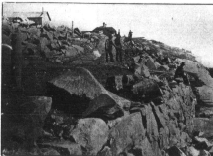
FORT FRANCES CANAL LOCK.
