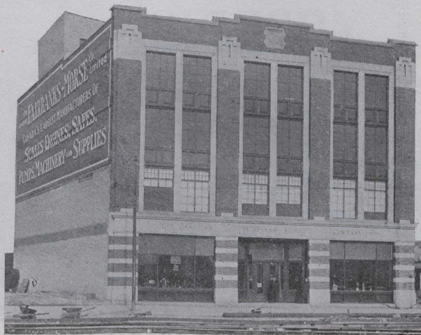
The New Fairbank-Morse Building, Saskatoon
