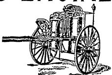
This machine is the most powerful fire fighter. It has two cylinders, 40 gallons capacity each. The combination of chemicals will not freeze, renders material with which it comes in contact non-inflammable, and will not cor ode when not in use. For full particulars, write to the Head Office of the Company at Kingston.
