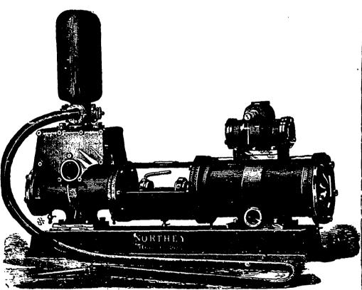
Ordinary Pattern Boiler Feed or Fire Pump. For Pumping Water against Heavy Pressure. Simple-Compact-Powerful.
