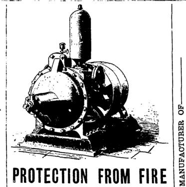
An Improved Rotary Piston Force Pump.
