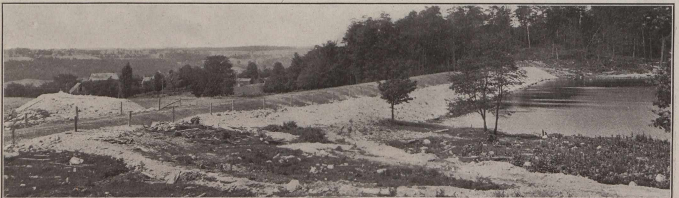
Fig. 5.—No. 2 Dam (earth filled) and Forebay.
