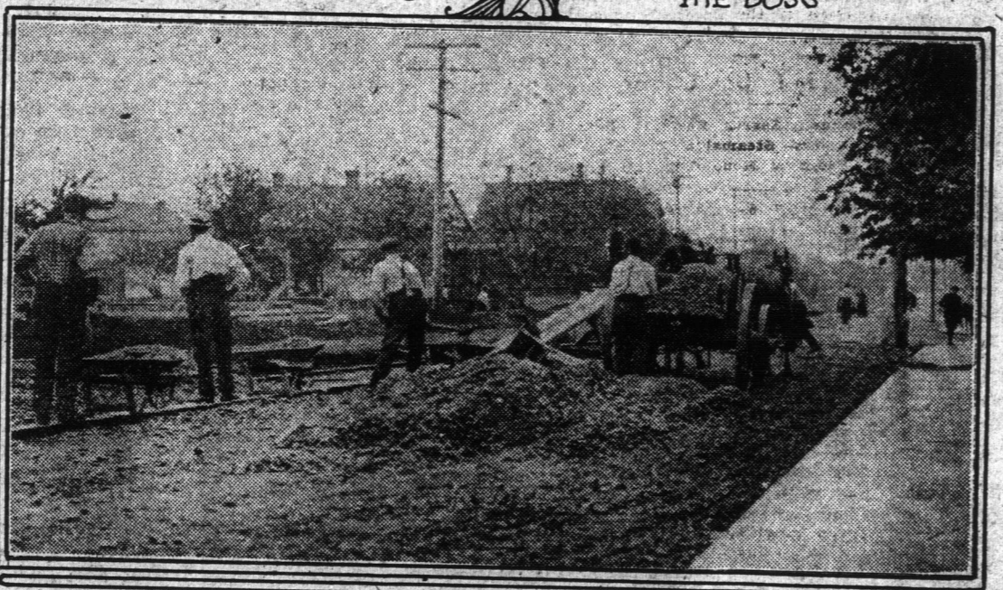
DUMPING THE CRUSHED ROCK
