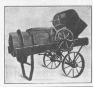
Specially adapted for Sidewalk and Street Work, and all classes of concrete work where a thorough mixture with but small capacity is required.
