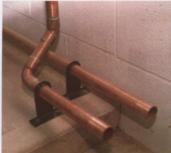
Pipe Stays, an innovative 'wall' support that speeds up the installation of pipe.
