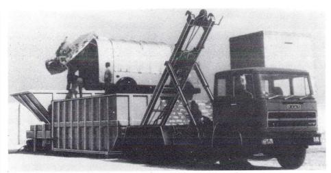
The Atlas Hoist and Body company's solid wastes transfer system.
