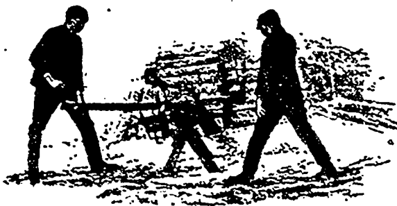
Working up the Wood-pile with a Cross cut Saw
