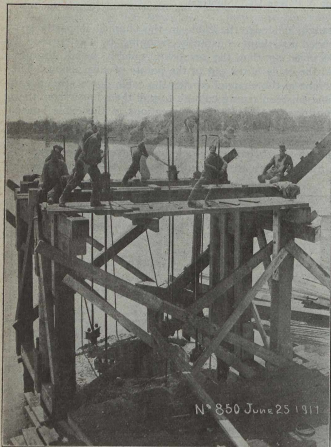
Lowering the Caisson—The Four Screws Were Turned Equal Distances Simultaneously
