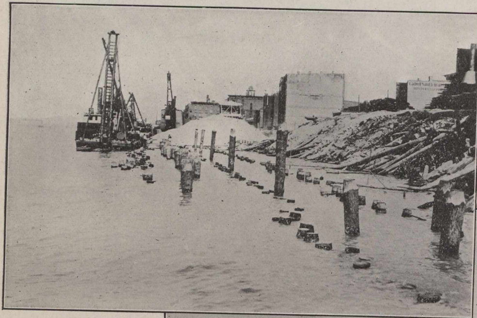
Rows of Driven Piling Before Framing; City of Detroit in Background of Lower View.
