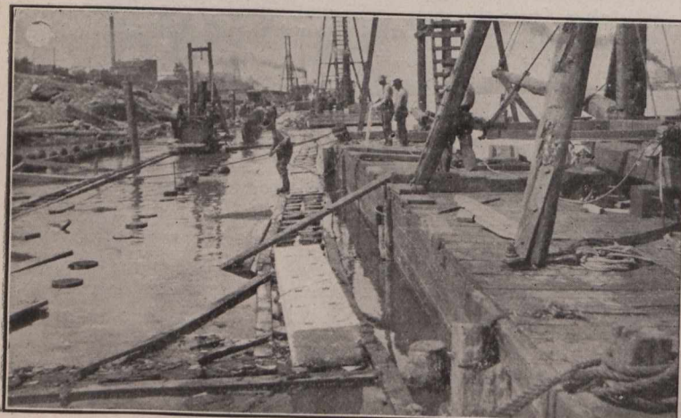
Anchor Piles Sheeted and Rotary Saw at Work on Rear Row of Bearing Piles.
