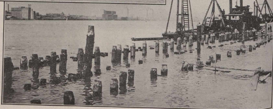
Rows of Driven Piling Before Framing; City of Detroit in Background of Lower View.
