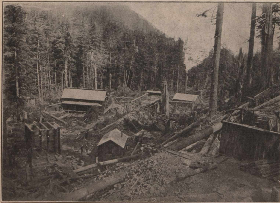
LILY MINE—FRONT VIEW OF No. 3 TUNNEL.
