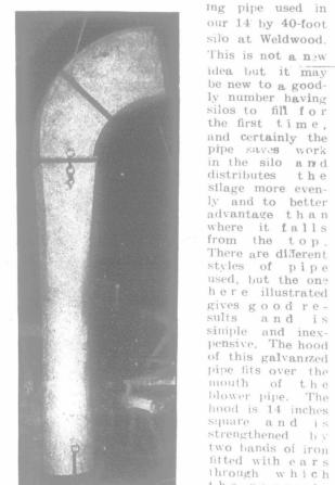
which the pipe The second length of pipe is suspended pass. tapers from square 'to round in shape, is eight inches in diameter and five feet long. All other lengths are five feet long. The pipes must fit loosely one into the other in order to give free oor young men it will be the defendin' of their
