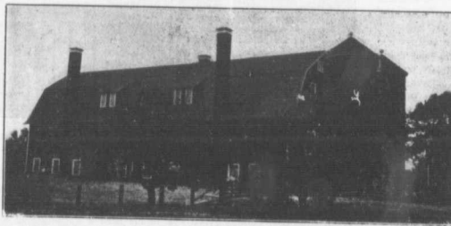
Mr. Dimick's Bontokoe Barn, Erected Especially to Take Care of His Reactors
