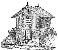
The engraving, reprinted from the Country Gentleman, represents the form of construction, when the lower part is built of stone and the upper of common vertical boarding. As the lower part is more than a foot in thickness, the timbers of the upper must be so constructed as to give an equal thickness, and to allow all the contents to settle alike. If, however, the whole is built of stone, this provision as to thickness is not necessary. It is hardly
