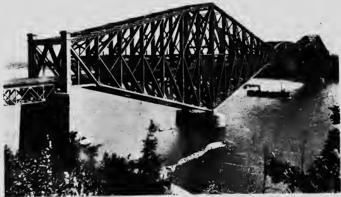
79 View of the Bridge from the North Shore
