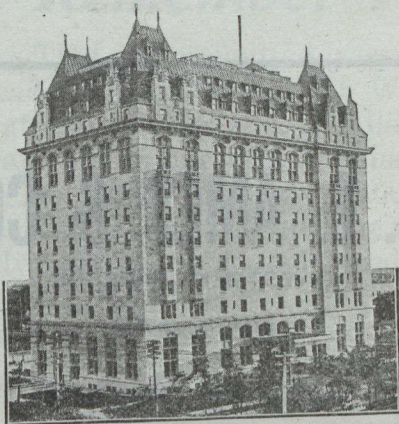
Fort Garry Hotel, Winnipeg. Arch: Ross & MacDonald, Montreal. El. Cont: L. H. Nielson Co., Inc. Pittsburgh.
