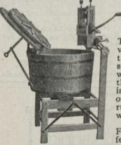
The tub rests and rotates on a set of perfected ball-bearings.
