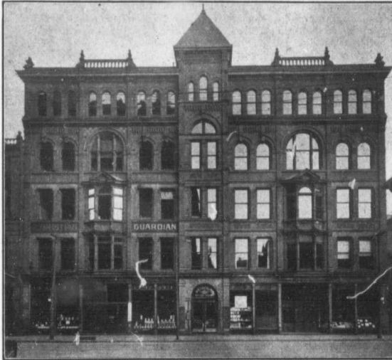
WESLEY BUILDINGS—AS THEY ARE NOW. RICHMOND STREET FRONT.
