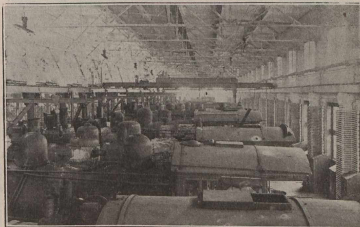
Fig. 4.—Erecting Shop Bay, Looking East.
