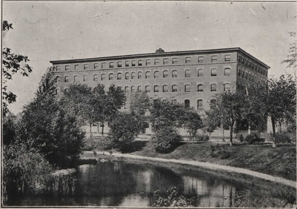
GOVERNMENT PRINTING BUREAU BUILDING, OTTAWA
