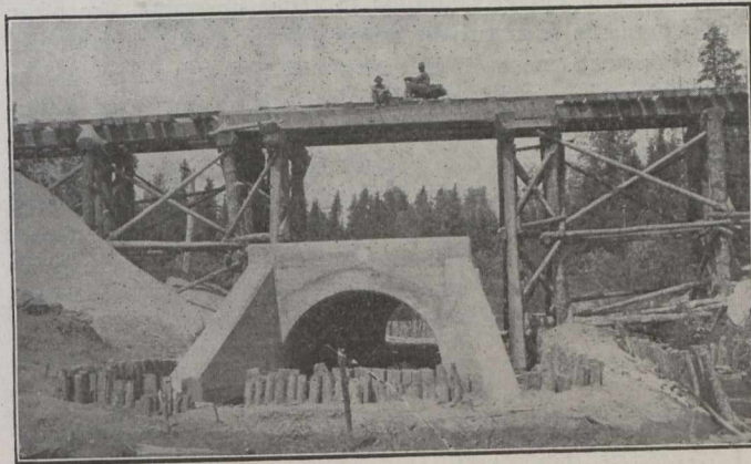
Fig. 10.—Typical Railroad Culvert in Earlier Stage of Construction.
