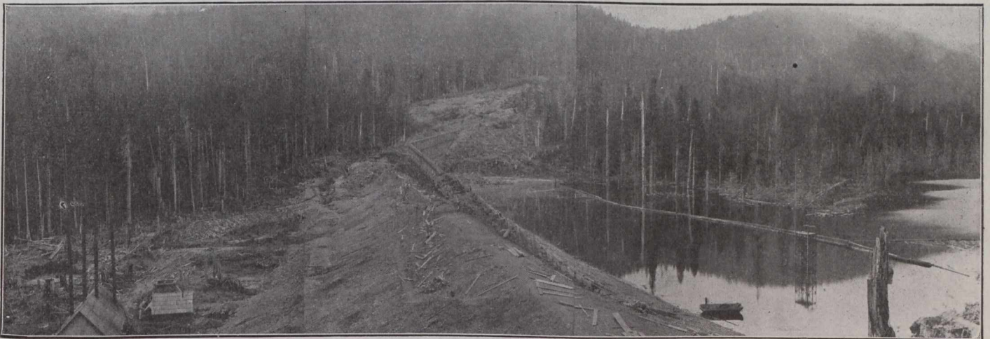
The Jordan River Development, Bear Creek Dam.
