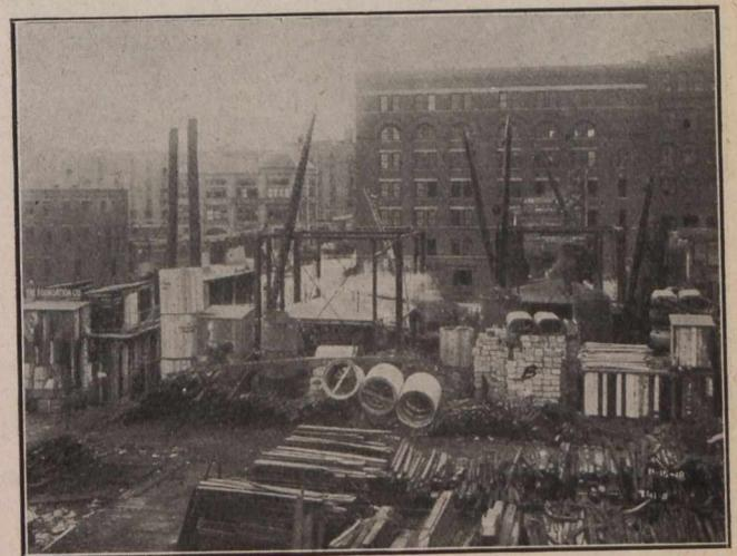
Fig. 2.—Showing Two Four-Masted Steel Derricks. Steel Forms used for Building up Cylinders—Collapsible Steel Shafts Inside of Steel Forms. Wooden Cofferdams, Used where Concrete Stopped Below Ground. Pile of Cast Iron Blocks Marked "B" Used for Weighting Down Caissons. Each Block Weighs 1½ to 2¼ Tons.
