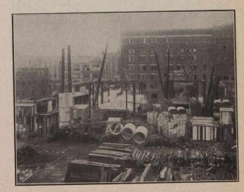
Fig. 2.—Showing Two Four-Masted Steel Derricks. Forms used for Building up Cylinders-Collapsible Steel Shafts Inside of Steel Forms. Wooden Cofferdams, Used where Concrete Stopped Below Cround. Pile of Cast Iron Blocks Marked "B" Used for Weighting Down Caissons. Each Block Weighs 11/2 to 21/4 Tons.
