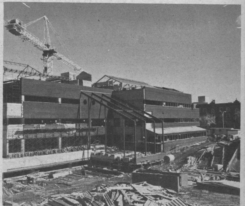
The new Agriculture - Forestry Center behind SUB
