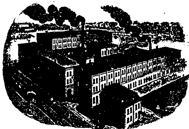
WORKS AT FORT WAYNE, IND.
