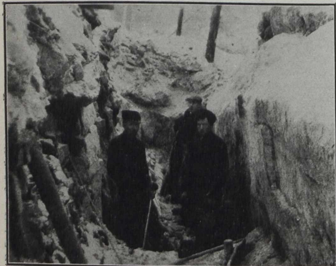
A 4-INCH VEIN OF COBALT ORE AT THE EVANS MINE.
