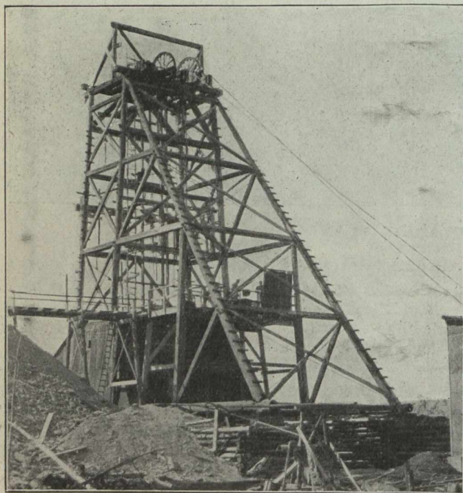
No. 2 Shaft, Dome Mine
