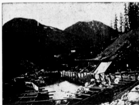
Sluicing out excavation for concrete dam.
